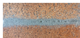
Insufficient paving gap showing Gap Sand sitting on top of pavers
