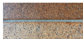
Correct paving gap showing bonded Gap Sand between pavers
